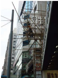
Worker erecting bamboo scaffolding in Hong Kong
